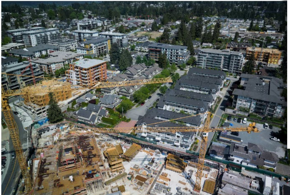
Cranes above a condo development and other housing projects under construction in Coquitlam, B.C. on May 16, 2023.
