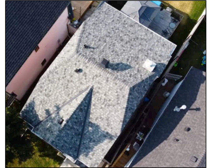
Class 4 IR Roof Cover – Calgary, 2022
