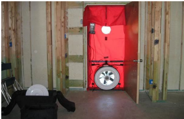
MID-STAGE BLOWER DOOR TESTING: Confirm air tightness targets
